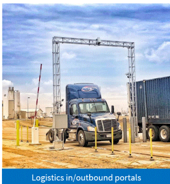
Logistics in/outbound portals
